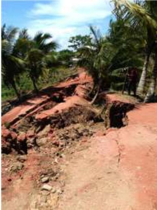
**Infrastructure damage from September 2018 7.4 Earthquake event at Erin, Trinidad showing significant land displacement**
